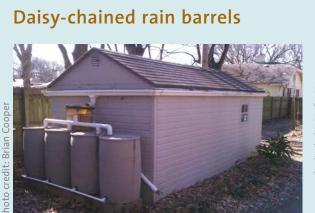
Brian Cooper daisy-chained four barrels together and added a feature to drain the first flush of water out the back.
