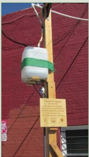
Water that flows out of the AC unit at Antigua coffee shop flows into this bucket, where it then flows by gravity into the garden.
