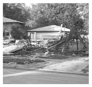
All that's left of a house that blew up because the gas was left on when the owner evacuated. The gas dryer floated up and severed its gas line, filling the house with gas. The security light timer turned on the lights at exactly 7:00 p.m. and BOOM! The explosion also totaled three other homes.
