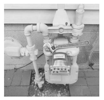
Keep a wrench close to your gas meter. *Caution*: After you turn the gas off, you should have the gas company turn it back on.
