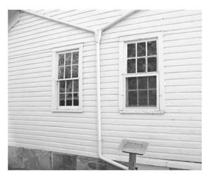
Amish home with gutters routed to basement cistern. A pump in the kitchen brings the water to the sink.
