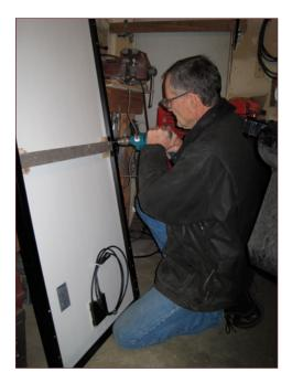
Drilling holes through photovoltaicpanel frame and horizontal aluminum support. Wood wedges hold aluminum support in place during drilling.
