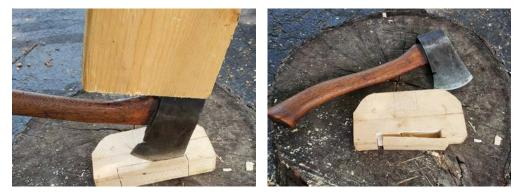
To split out the waste, I start with the upper corner of my hatchet and strike firmly with a scrap of wood. This construction lumber is soft, so the edge should plunge right in. After I've worked along both sides of my line, the waste comes right out.
