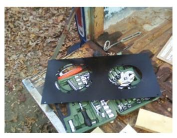
Once the plate arrived, I measured it and built a frame of scrap 2×4. The plate measured 12×24 so I cut two 2-foot lengths of 2×4 and 2 9-inch lengths. After screwing them together, it made a perfect frame.
