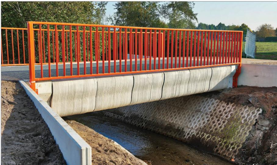
**FIGURE 2.7** – The world's first 3D printed bridge. Marczoutendijk.
